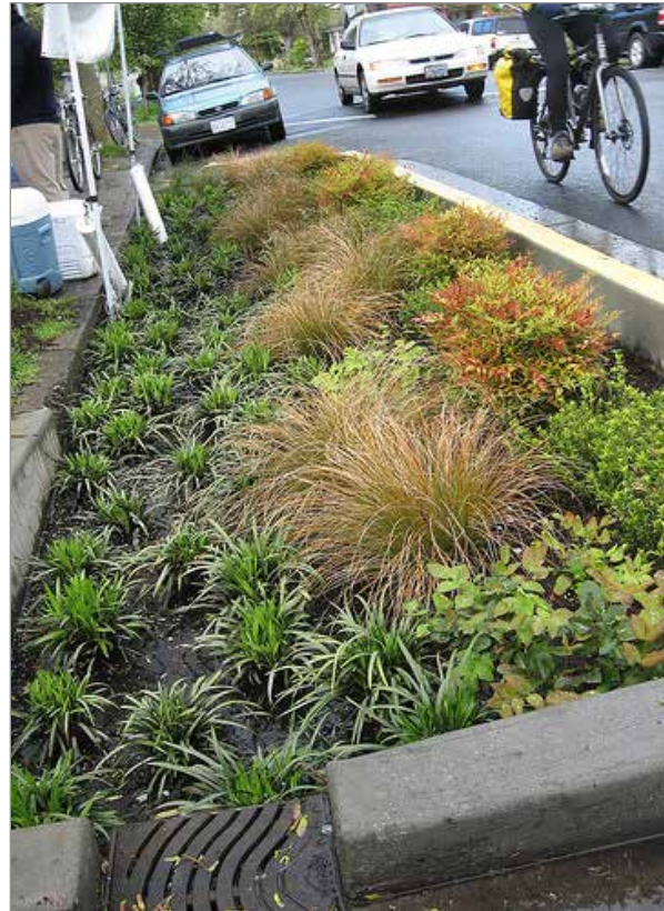
Stormwater runoff can be naturally filtered by using permeable pavers or by draining to landscaped areas as shown above.
