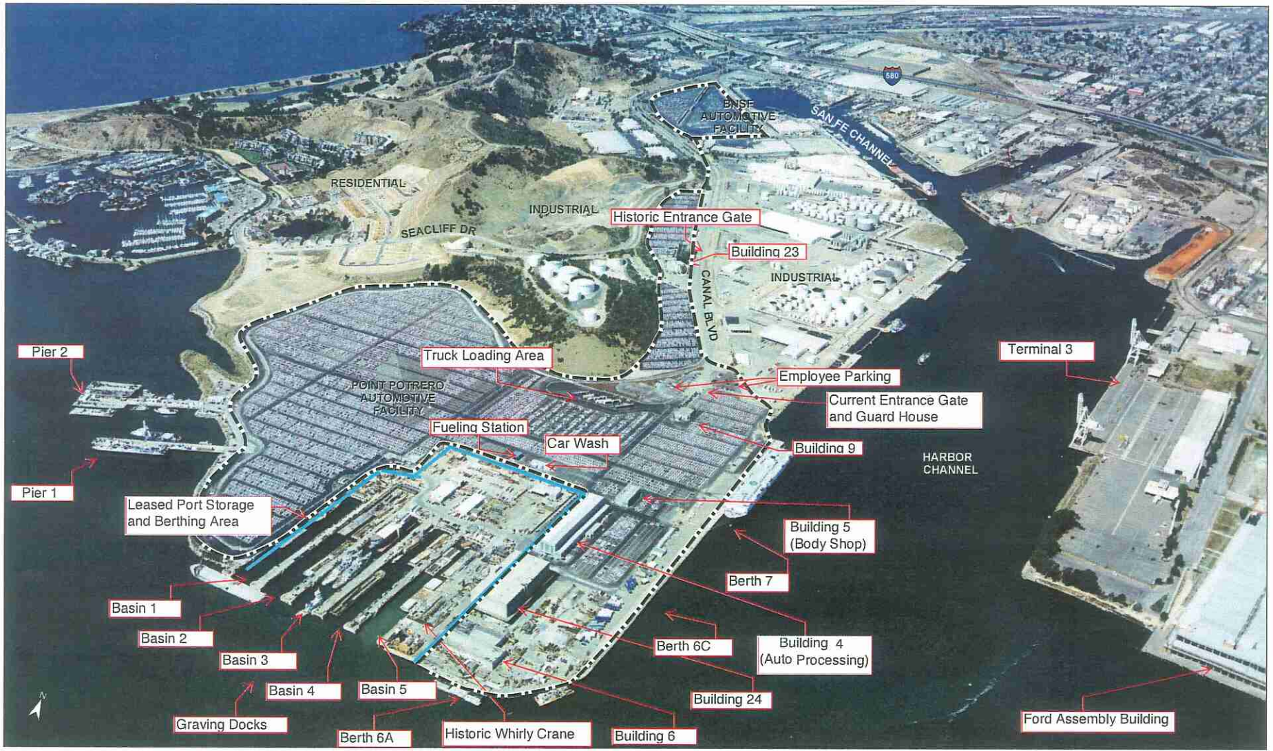
Figure 2 Overview of Existing PPMT Facilities
