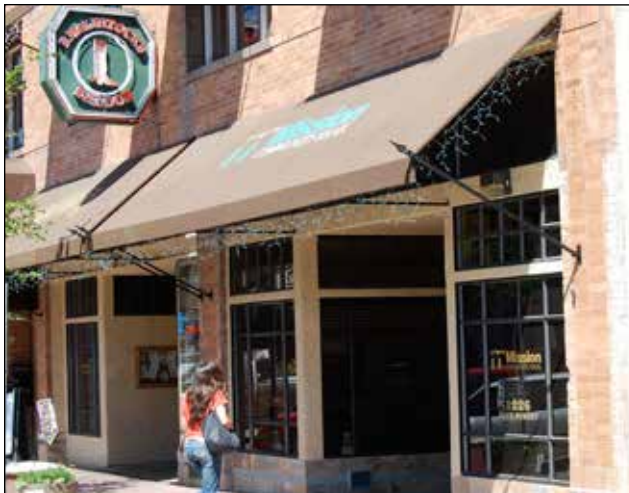
Awning with decorative supports and open end.
