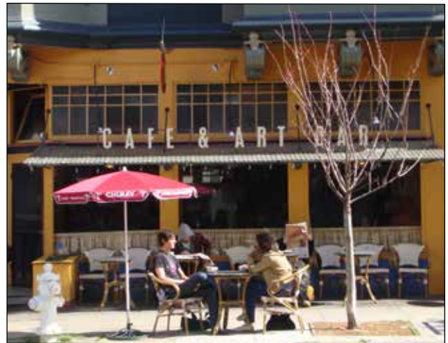
Projecting signage on a metal awning.
