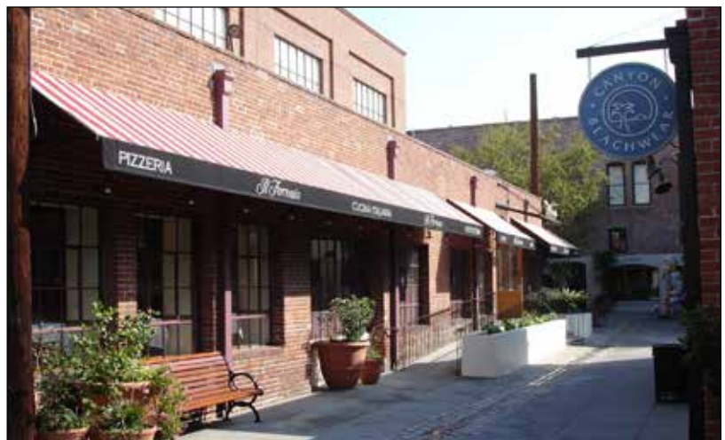
Series of awnings along a frontage.
