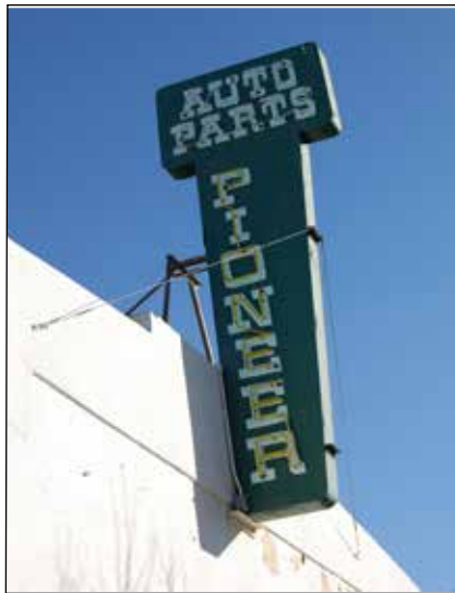
Marquee sign projecting above parapet.
