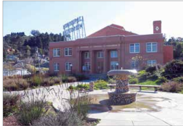
The Plunge (after renovation)
