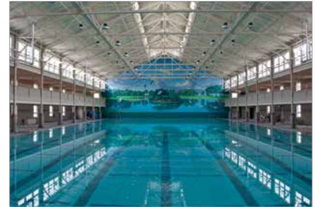
Inside the Plunge (after renovation)
