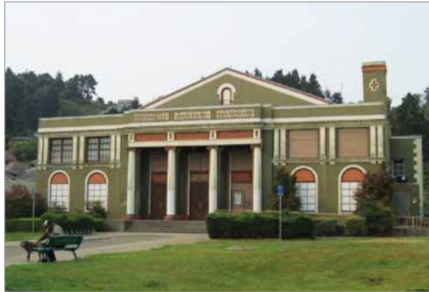
The Plunge (before renovation)
