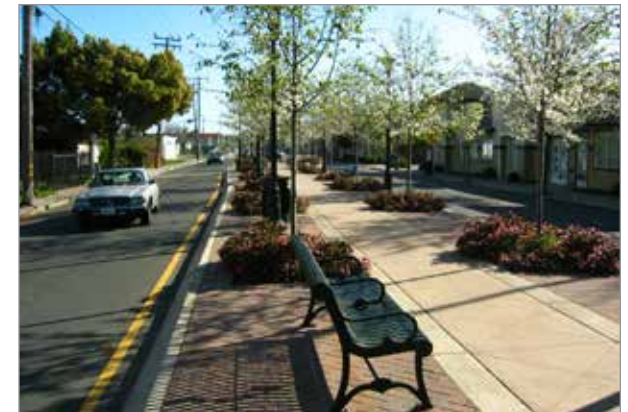
Streetscape improvements can transform automobile-dominated thoroughfares into complete streets that support all modes of travel and improve safety.
