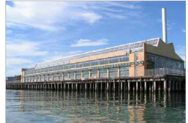
The redevelopment of the Ford Assembly Building has brought economic opportunities to Richmond.
