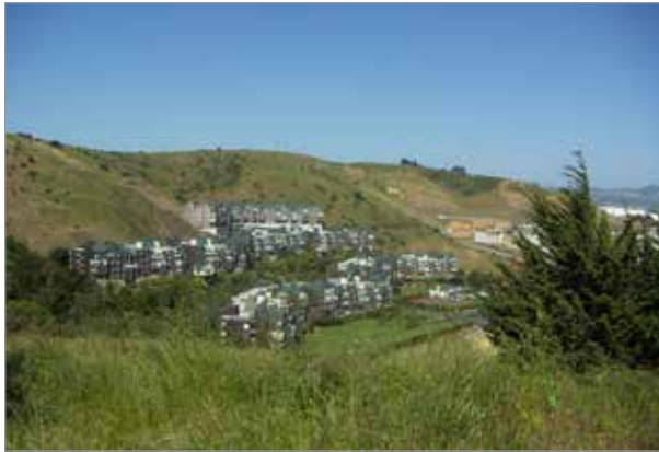
Effective measures to prevent landslides are essential when developing on steep slopes.
