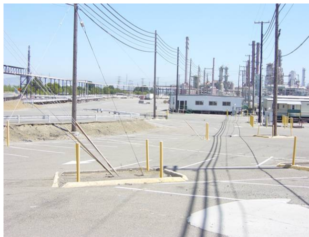
Figure 3-6 The "Y" area of the Refinery
