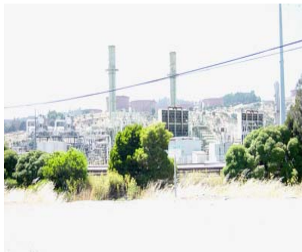
Figure 3-11 Existing CoGen Units
