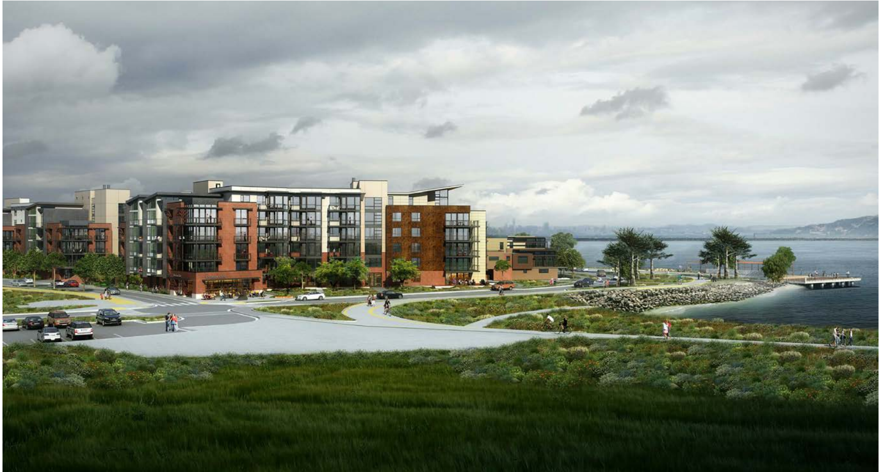
VIEW OF BUILDING 1 FROM WEST
