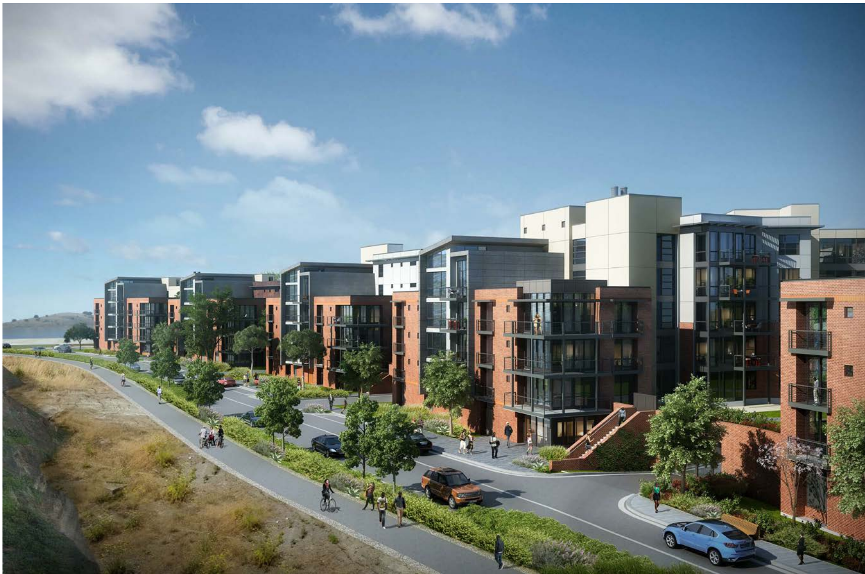
VIEW ALONG BRICKYARD COVE ROAD
