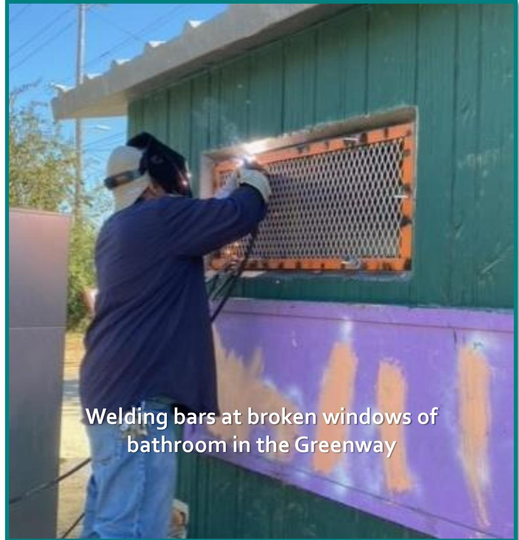
Welding bars at broken windows of bathroom in the Greenway
