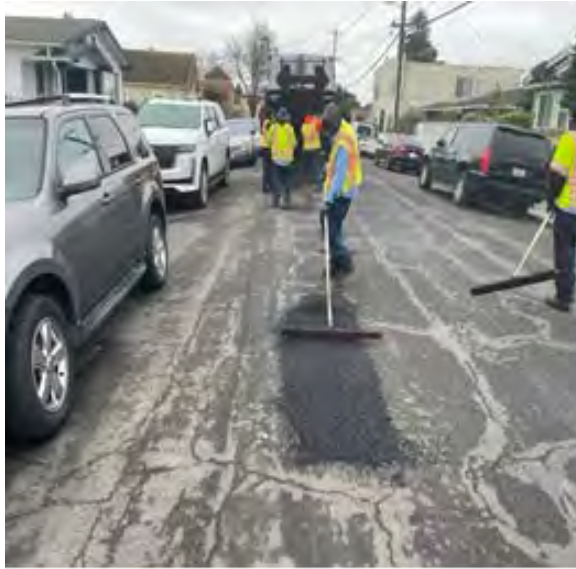
Hot mix patching at various locations
