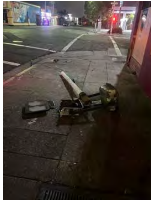
Traffic signal knockdown on MacDonald Ave
