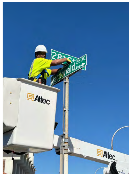
Installed name sign at MacDonald Ave and 28th Street
