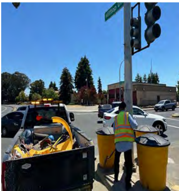
Installed new Crash Barrels on Hilltop Drive
