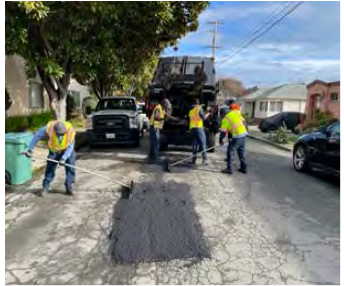
Hot mix patching at various locations
