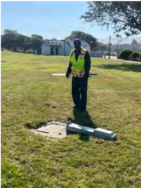
Installing power pedestals at the Marina
