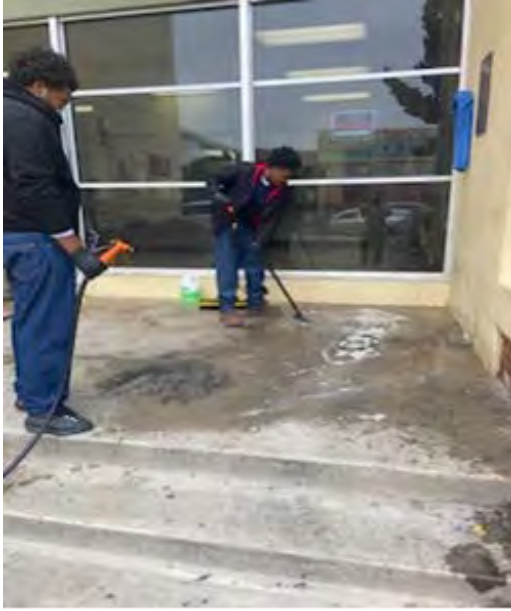
Cleaned entrance of Recreation Complex
