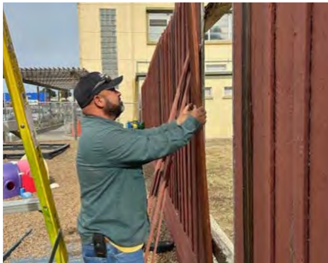
Fence repair at Recreation Complex
