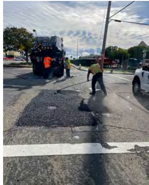
Pothole patching on Barrett Ave & hot mix at Marina Way South
