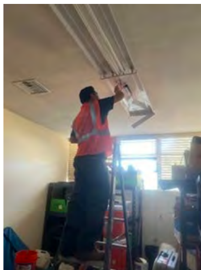
Lighting repairs at Memorial Youth Center
