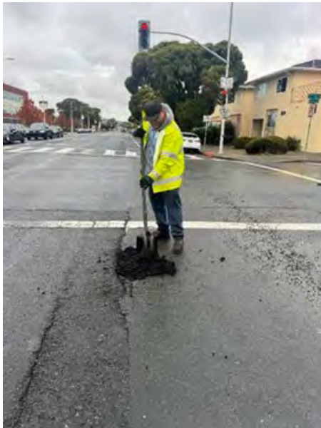
Pothole patching on Barrett Ave & hot mix at Marina Way South
