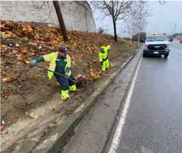
Removal of debris from v-ditches
