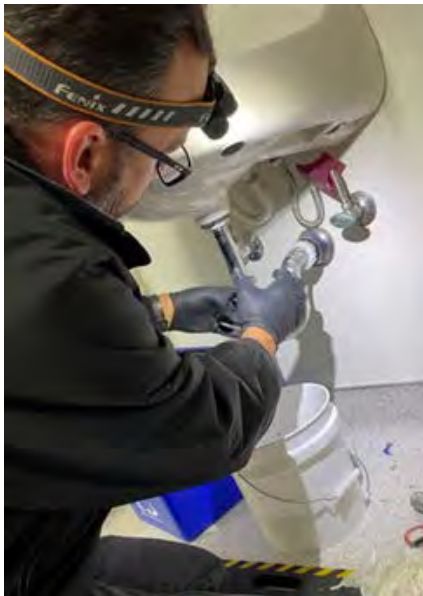
Drain repair at Police Department locker room
