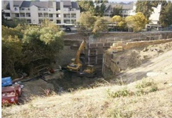
**Culvert Headwall area:** The culvert headwall area has been dewatered and shoring has been installed to protect the Creek View Condominiums property, visible in the background.
