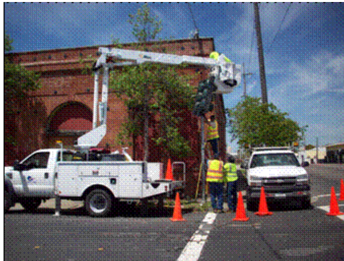
Intersection of Harbour Way and Ohio Avenue
