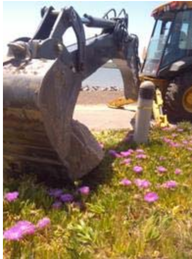
Marina Bay lighting repairs
