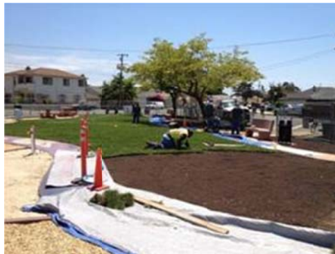
Solano Play Lot Sod Installation
