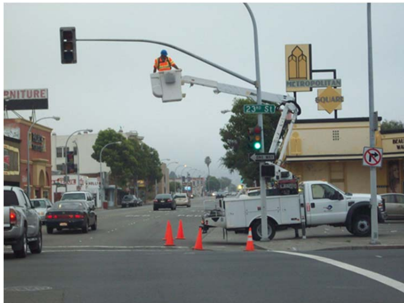
Replacing Green Light on Macdonald Avenue and 23 rd Street
