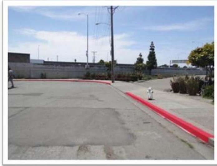
Curb Maintenance on Wall Avenue
