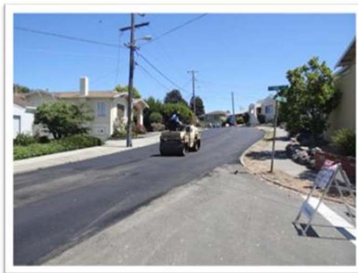
Paving on Ventura Street
