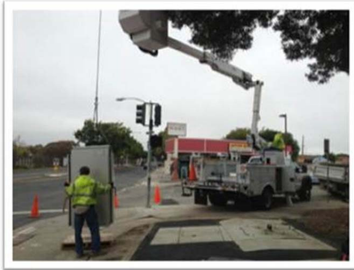
Traffic Signal Cabinet Installation on So. 47 th and Carlson Boulevard
