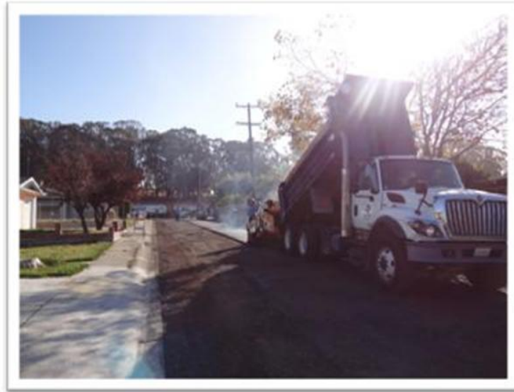
Paving on McGlothen Way
