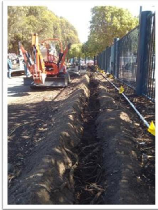
Meeker Trail Landscape Rehabilitation
