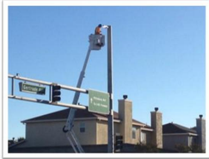
Repairs to Safety Lights
