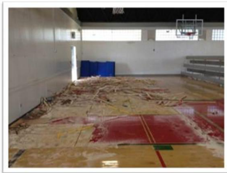
Repairs at Richmond Recreation Complex
