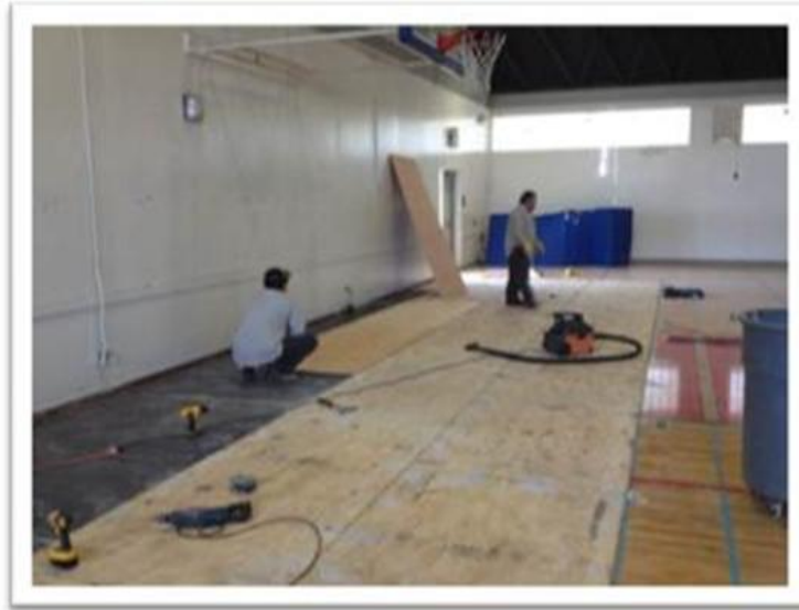
Repairs at Richmond Recreation Complex
