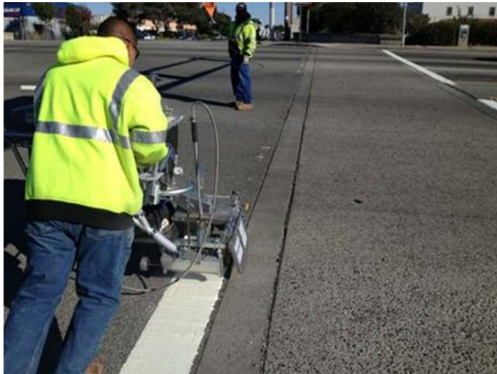
Placing Thermoplastic Crosswalk
