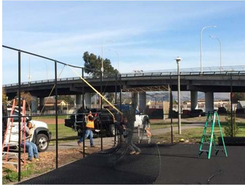
Fence Installation at Lucas Park
