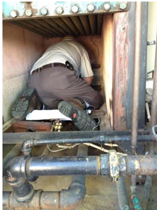
Boiler Repairs at Employment and Training
