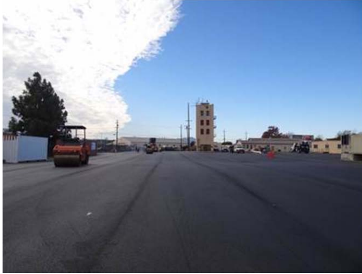
Paving at the Fire Training Center
