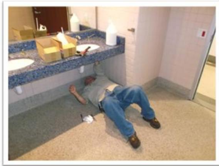
Soap Dispenser Replacement
