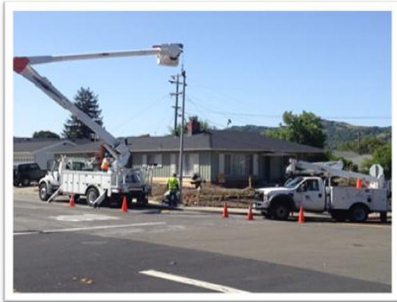
Pole Replacement on Morwood Drive and May Road
