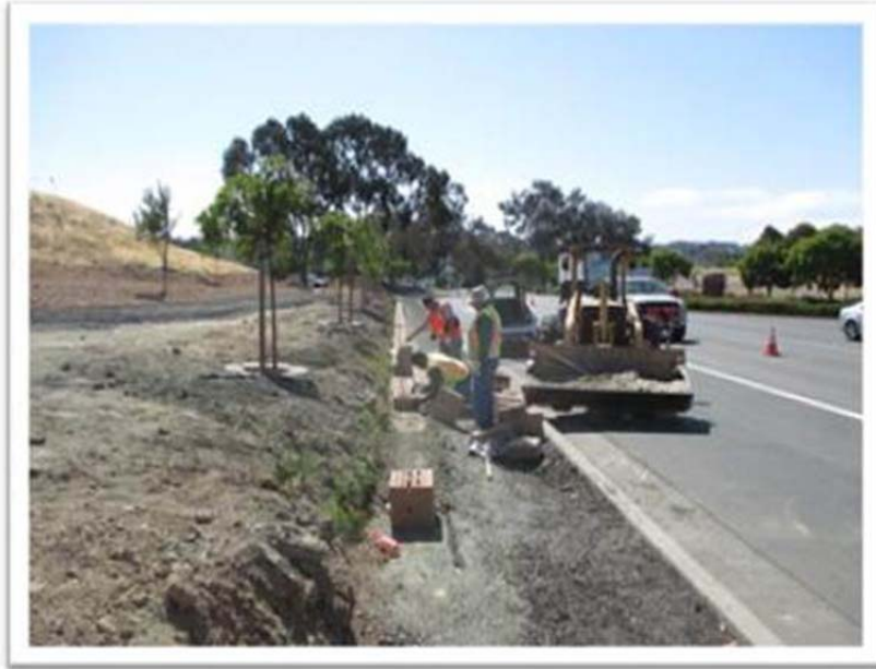
Richmond Parkway Pathway Project
