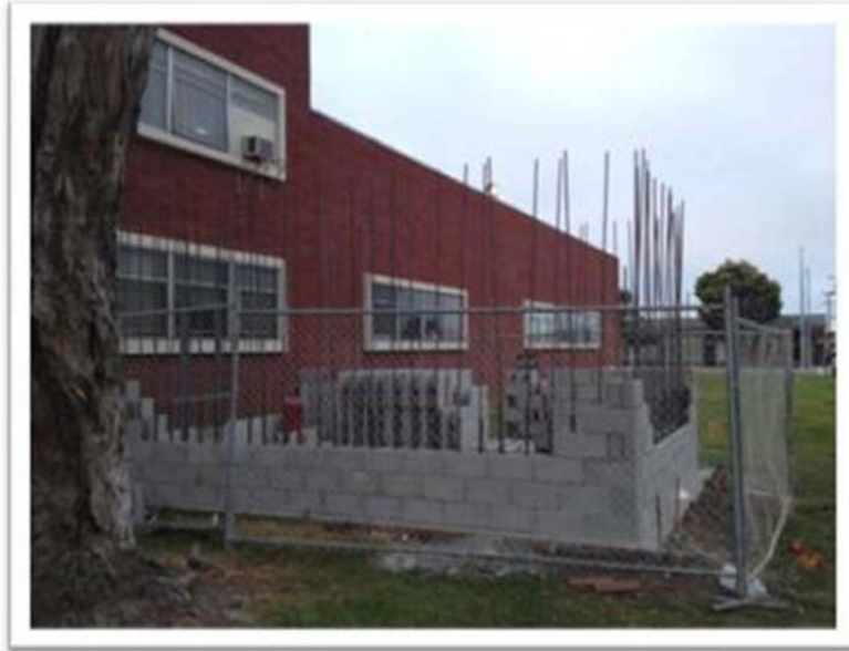
Construction of Emergency Generator
