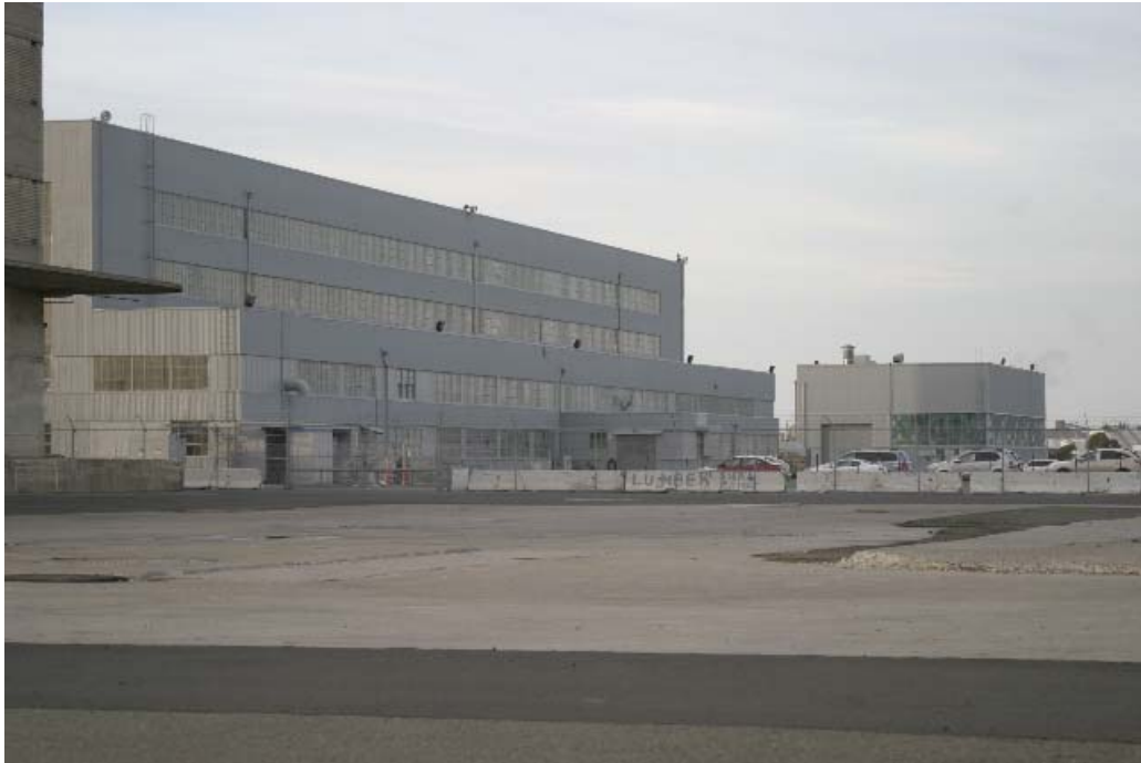
a) Buildings 4 (historic machine shop, foreground) and 5 (historic forge shop.)
