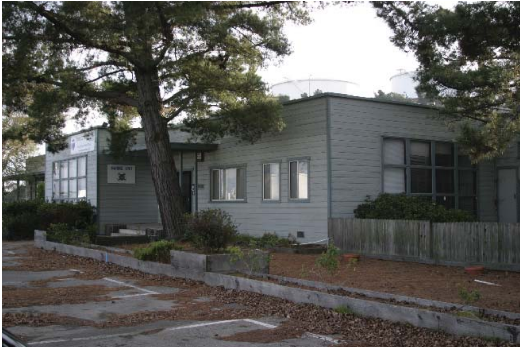
b) Building 23, the historic cafeteria adjacent to the historic entrance to Kaiser Shipyard No. 3.
