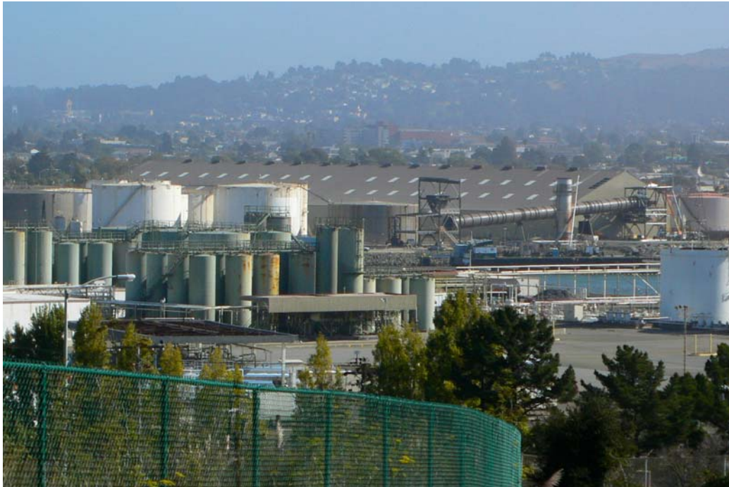
a) A partial view of the Conoco/Phillips and Kinder Morgan industrial properties located on the east side of Canal Boulevard.
