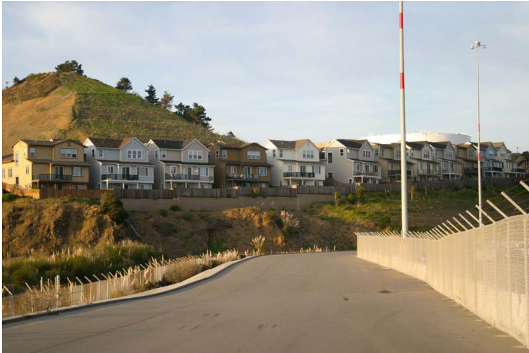
a) Homes in Seacliff Subdivision overlooking the western end of the PPMT.
