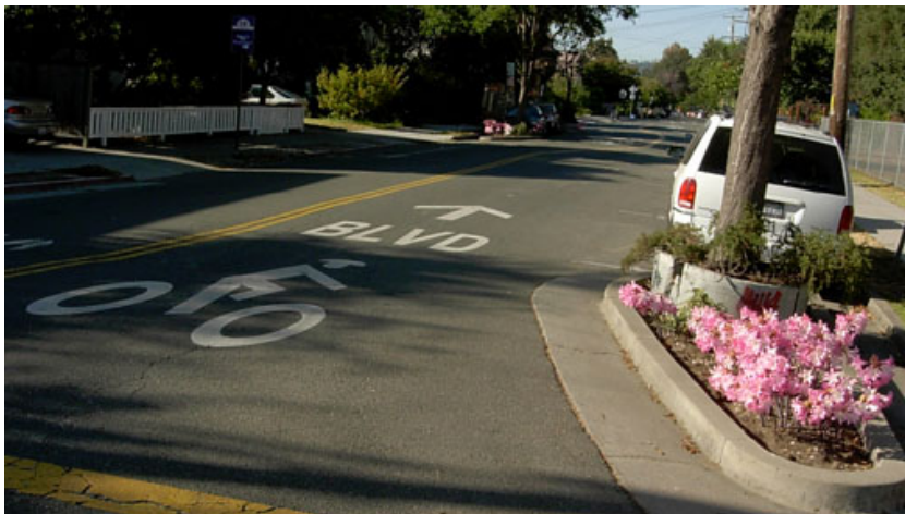
Bike Boulevard in Berkeley, California
