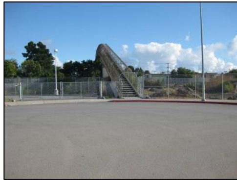
The 33 rd Street Bridge provides non-motorized access over the BART tracks
